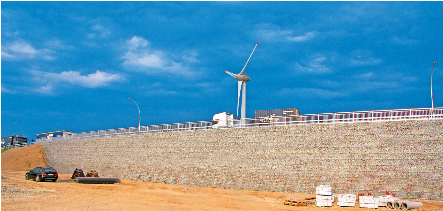
Retaining Walls in Altenwerder
