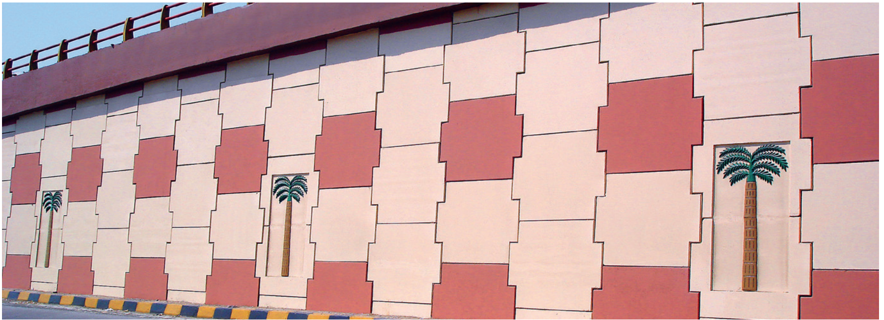
Navghar Flyover, Mumbai International Airport Mumbai, India ►
