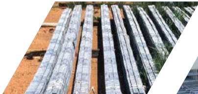
Steel strips reinforcement
