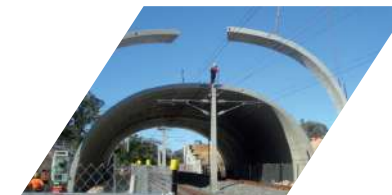
Installation of TechSpan®, Mandurah - Australia
