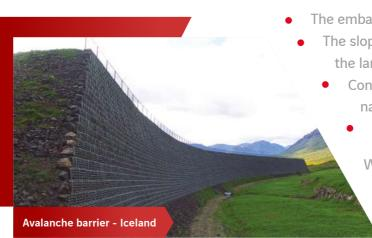
The embankment slope can be steepened up to 90°;
